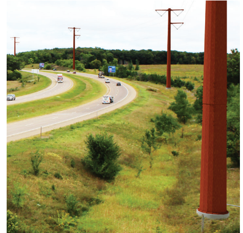
This simulated image demonstrates what a new 345-kV line could look like.
