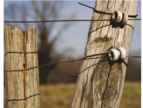
Electric fences are specially insulated from the ground and can pick up an induced charge from transmission lines.
