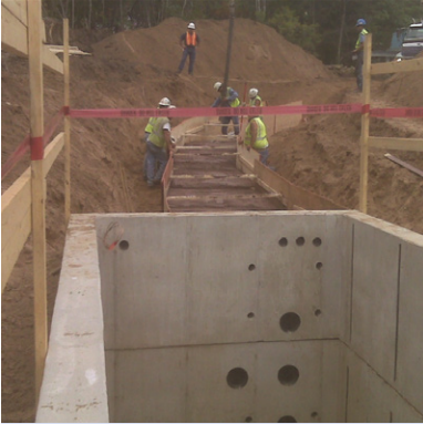
Crews work on an underground duct bank extending from a typical 8'x8'x24' vault.
