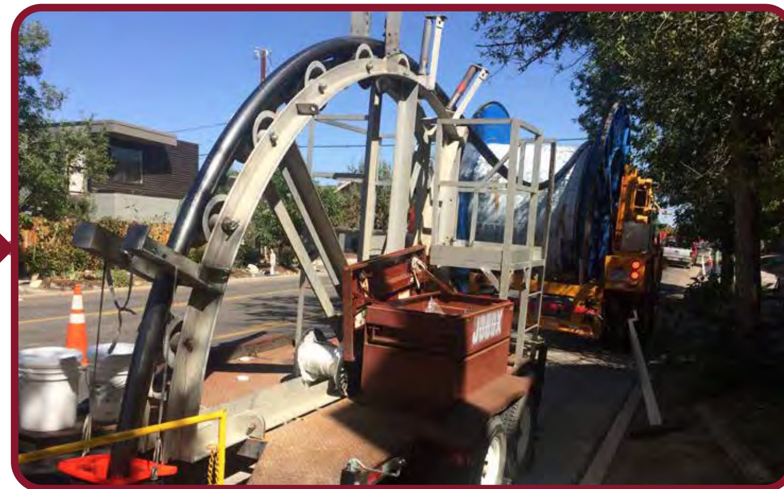
Install electric cable system
