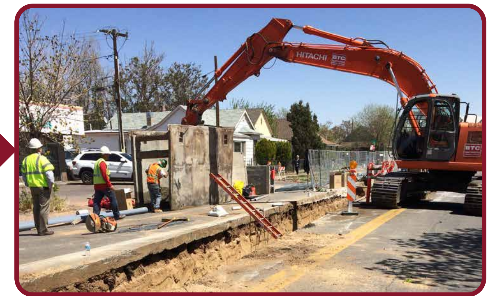
Install trench boxes and conduit
