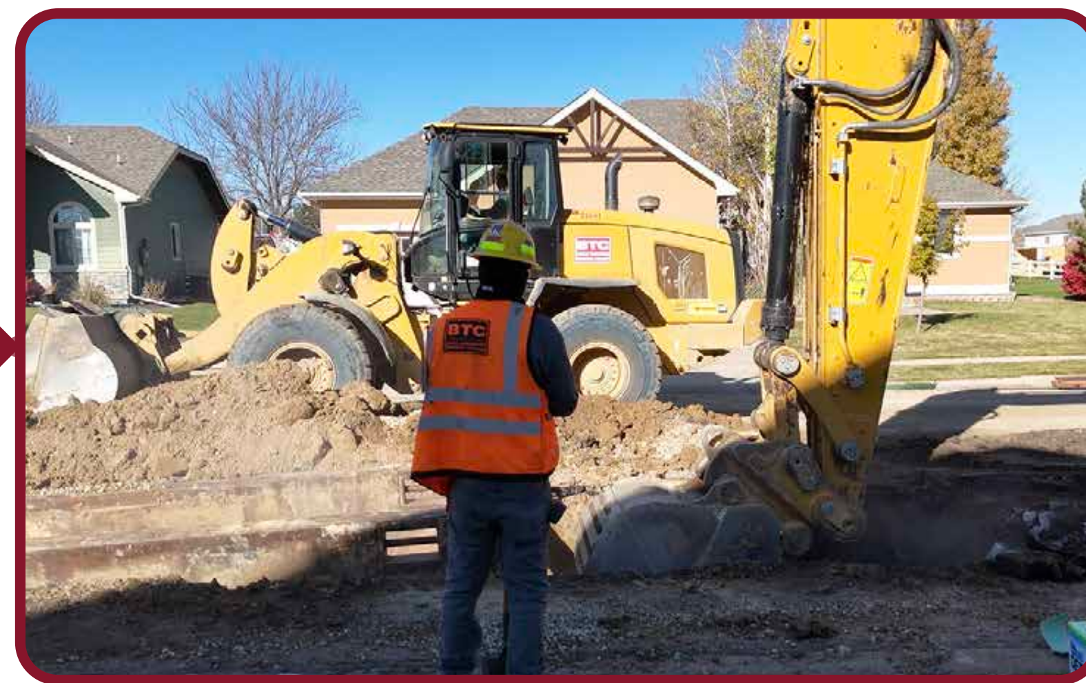
Remove pavement and excavate trench
