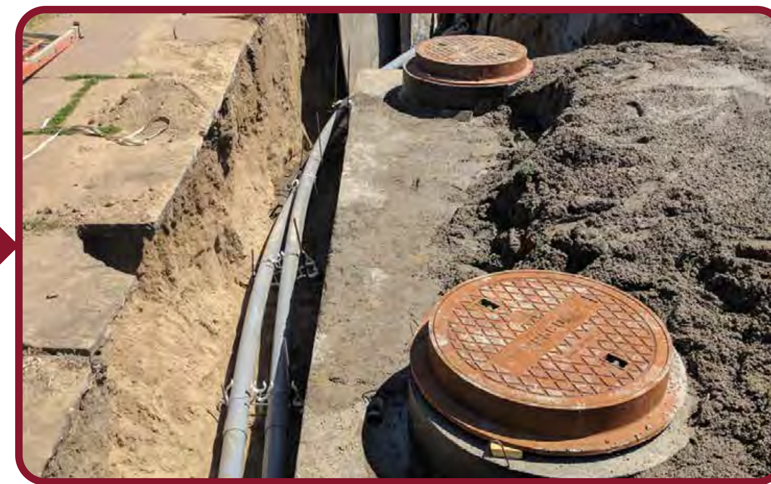
Install precast splice vaults with manhole covers
