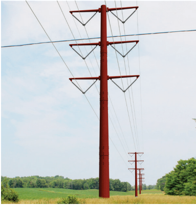
Simulated image demonstrates a 345-kV transmission line 'double-circuited' with a 1150kV transmission line.
